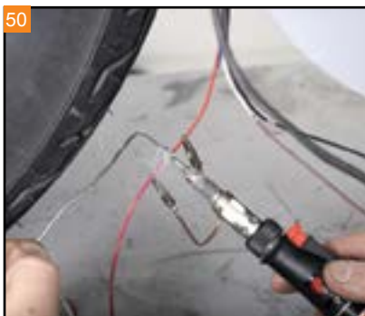
50 Extend the wires from the right side Wedgy Light. Ensure all the solder joints are covered with shrink wrap individually, then all the wires together.
