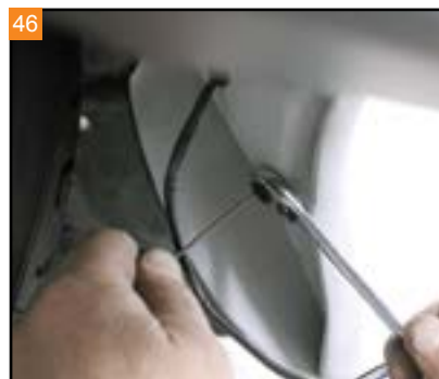
46 Hold the stud in place while tightening the lock nut on the backside with a 5/16" wrench.
